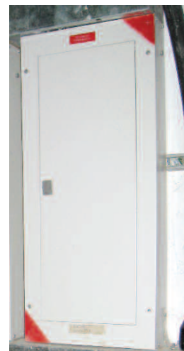
MCB boards inside the main-switch room
