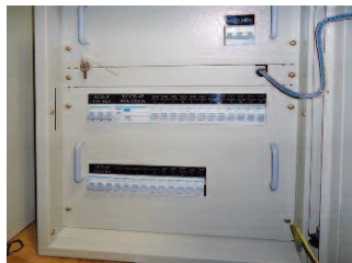
enclosure with MCB and RCCB
