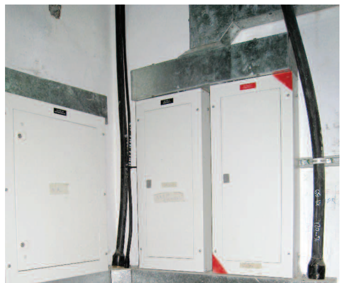
MCB and MCCB boards inside the main-switch room
